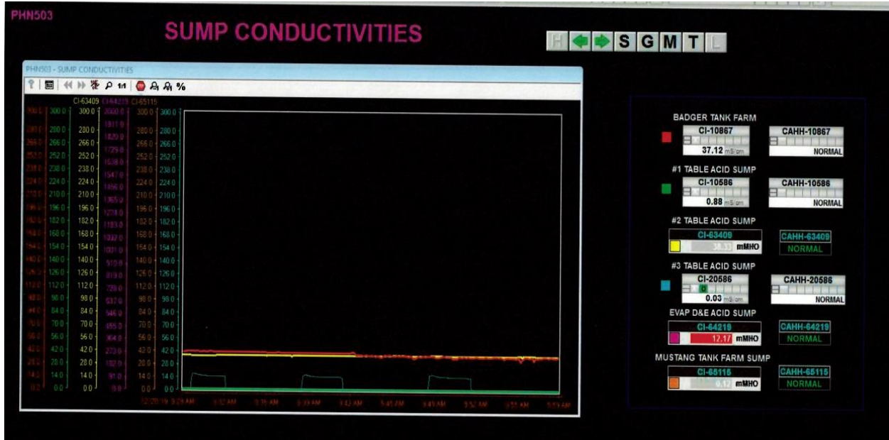
Figure 5: Example of Operator Monitoring Graphic
